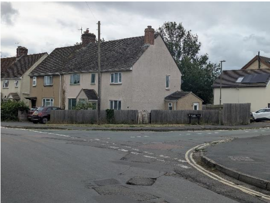
Figure 86: Poorly maintained dropped kerbs, and lack of tactile paving at junction of Back Lane and Spareacre Lane
