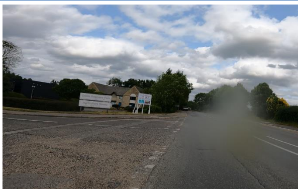
Figure 76: Wide junction mouth, at Oasis Business Park, with no dropped kerbs or tactile paving
